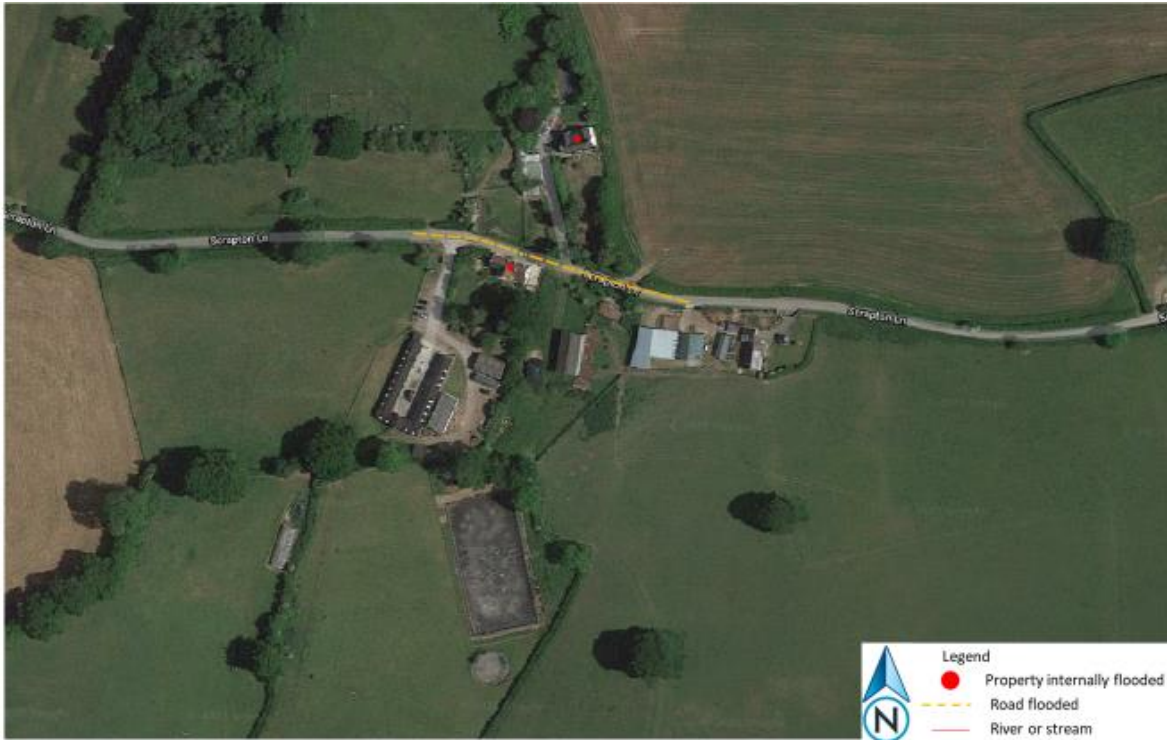
Figure 32: Flooded properties and road damage in Scampton Lane
